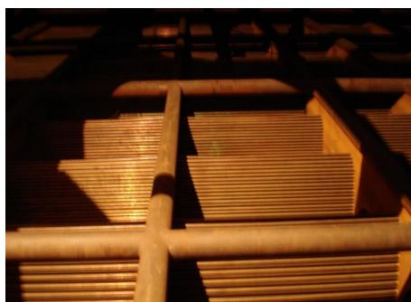
**Fig. 1.** Tubular stack of heat exchanger pipes.
