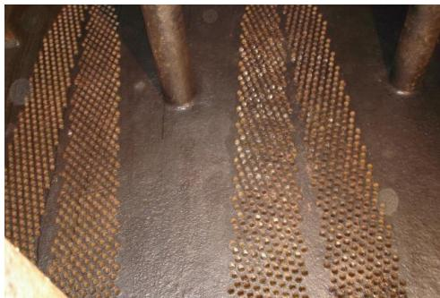
**Fig. 3.** Back wall tubular plate and heat exchanger pipes arrangement.
